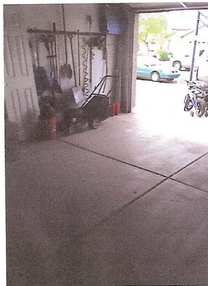
Garage – Southwest After
